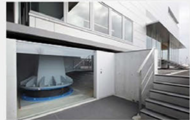
Seismic isolation system
