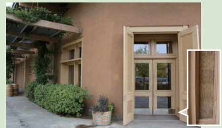
Building constructed with rice straw in the walls
