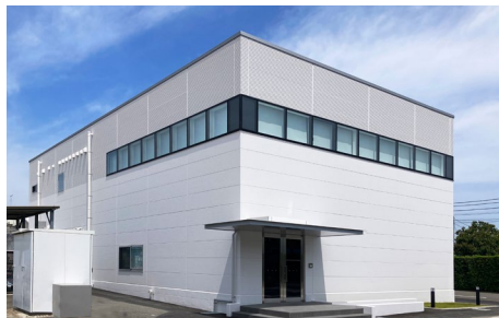
Otsuka Group Energy Management Building
