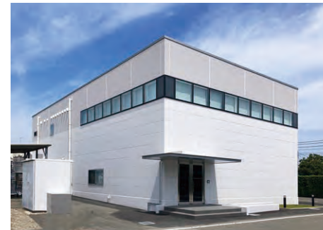
Otsuka Group Energy Management Building
