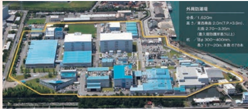
Otsuka Pharmaceutical Factory: Full-circumference seawall built against tsunami
