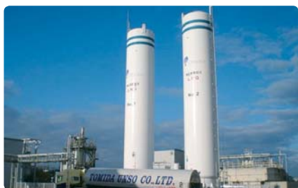
Matsushige Plant of Otsuka Pharmaceutical Factory
