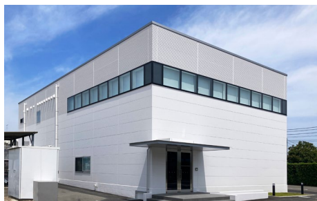
Otsuka Group Energy Management Building
