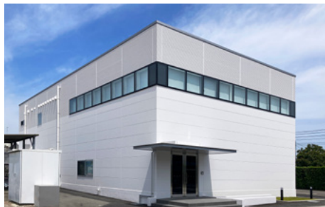
Otsuka Group Energy Management Building
