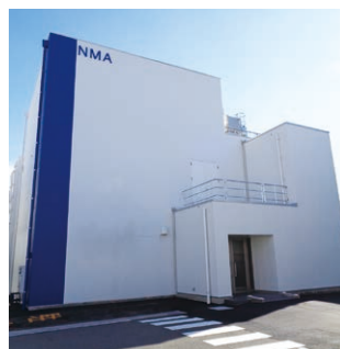
SynCrest Inc., a joint venture with Yokogawa Electric Corporation (a plant for the manufacture of bulk pharmaceuticals for medium-molecule drugs)
