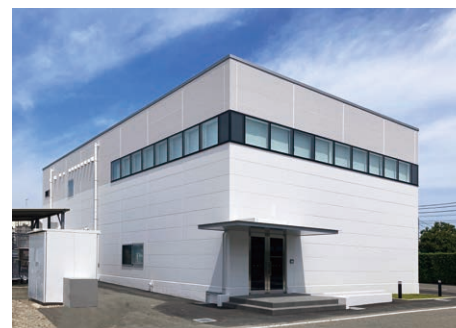
Otsuka Group Energy Management Building
